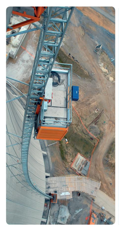
Additionally the power supply cable had to be specially installed. A cable trolley was placed underneath the hoist cage so that the ground station was slightly elevated to accommodate this. Due to the changing inclination throughout the entire lift cable guides disruptions may have occurred. To overcome this anticipated problem the cable guides were manufactured with special rollers so that the cable tension was minimised.
