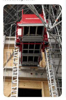
HVB Tower is mushroom shaped. The tall building stands on a narrower foot which is 21 meters high. The shape of the building placed a special requirement for the mast anchoring of the hoist. From the ground level there were 23 meters of empty space above, before the first available anchoring could be placed.
