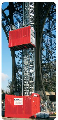
n spring 2008 Scanclimber's partner Sky Accès in Paris was given the order for the delivery of a building hoist type SC2032F for the transport of both passengers and material which should be erected at one of France's most famous monuments: the Eiffel Tower.
