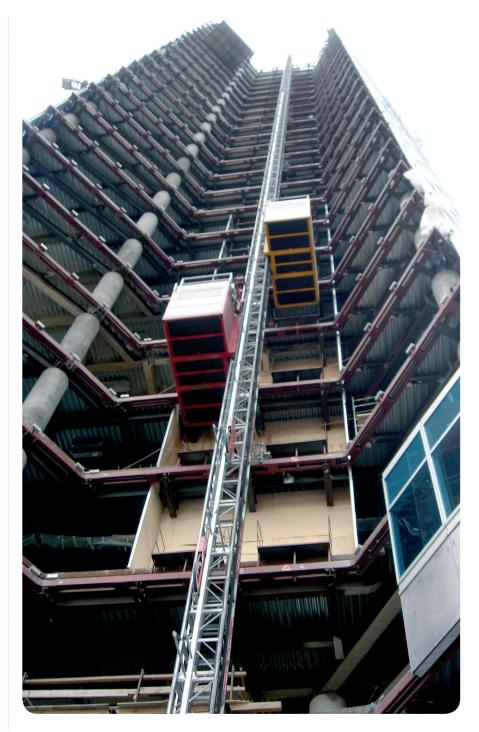
as possible. For this purpose the hoist was equipped with special anchoring which enabled a vertical anchoring distance of 21 m installation of the mounting plates onto the building was agreed upon with the steel construction in order to place the anchoring in an area where sub-
