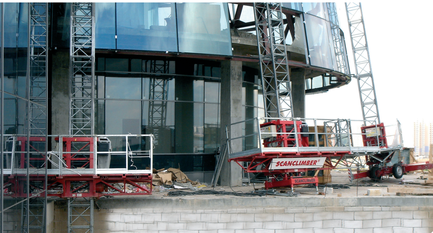
SC4000 work platforms on mini chassis and on wheel chassis mounted in an angle according to the wall
