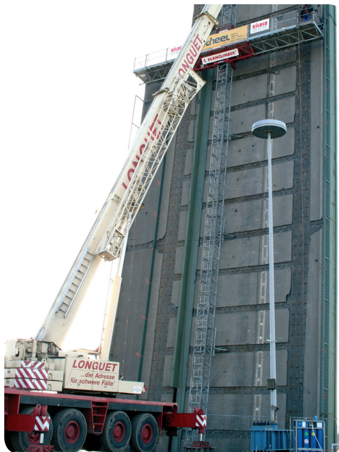
SC4000 lying with 7° slope used as single mast transport platform
