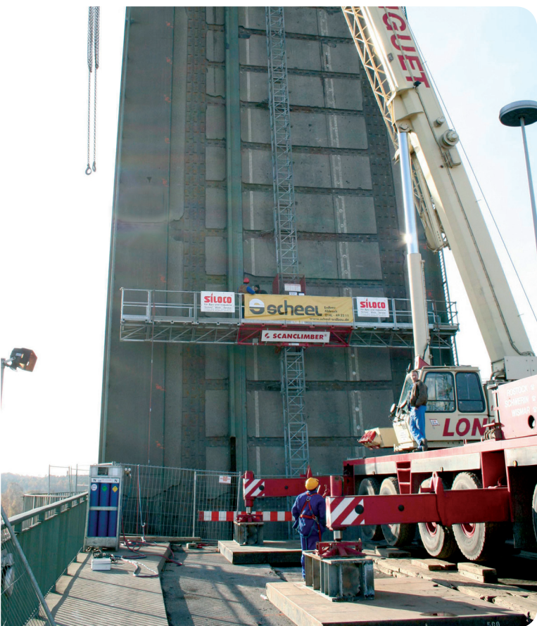
SC4000 lying with 7° slope used as single mast transport platform
